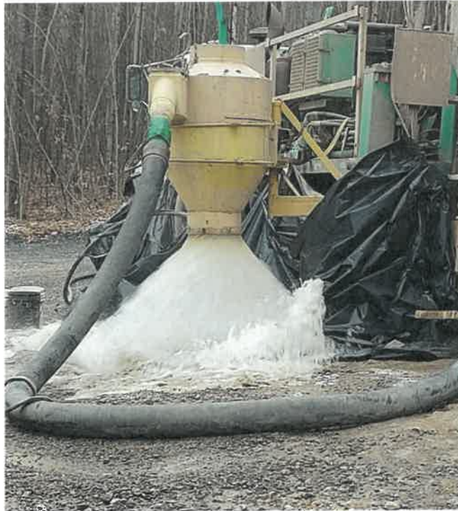
Discharge of over 700 gpm during development of Well PW-1 that HSA located for the City of Plattsburgh, New York
